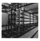
The RO water is blended with a small portion of filtered water to reduce the corrosiveness of the water and improve taste. Pure RO water also tends to have little taste. Blending water back adds the minerals required for the taste many consumers desire and is
