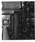
are so small however, that dissolved solids in the water (radium, hardness, sulfates, etc.) are not able to pass through the membrane and are discharged in a reject stream. The membranes remove 95 to 99 percent of all contaminants found in Sherburn's water including hardness and sulfates. This reverse osmosis process is the opposite of the osmosis process that occurs in nature when clean water passes through plant membranes into the roots.
